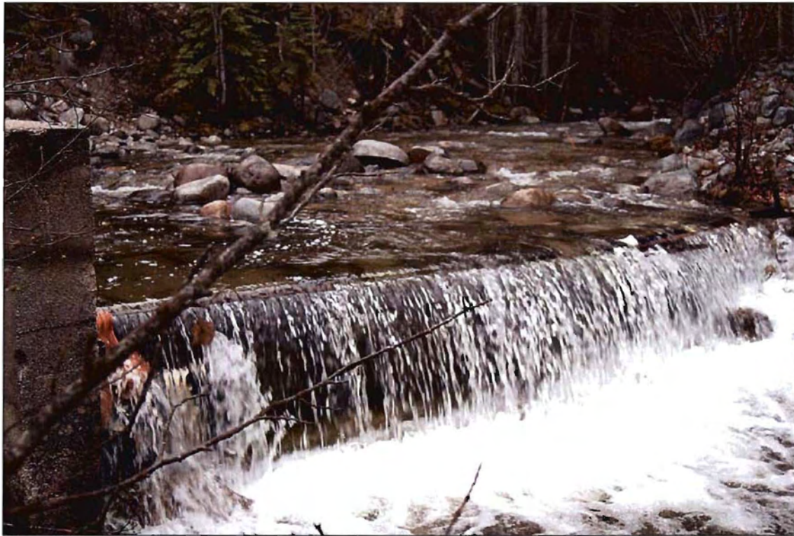
Example of fish passage barriers that are found on most streams in the watershed. Photo by Kevin Bradford.
